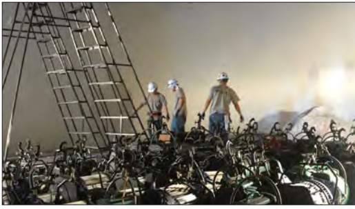
Specialty contractors work around studio lights.
