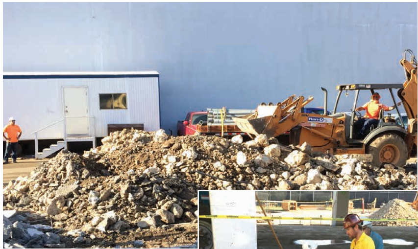
Above: Workers remove concrete from the existing building of the former KFVE Newsplex.
