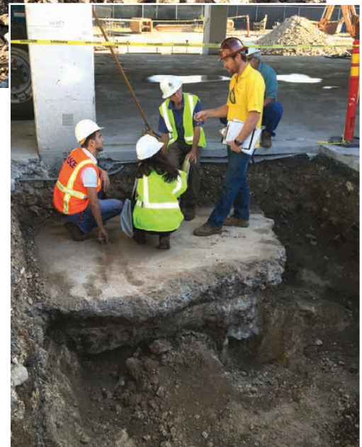
Workers meet in the pit that will become an elevator in our NEW HOME.
